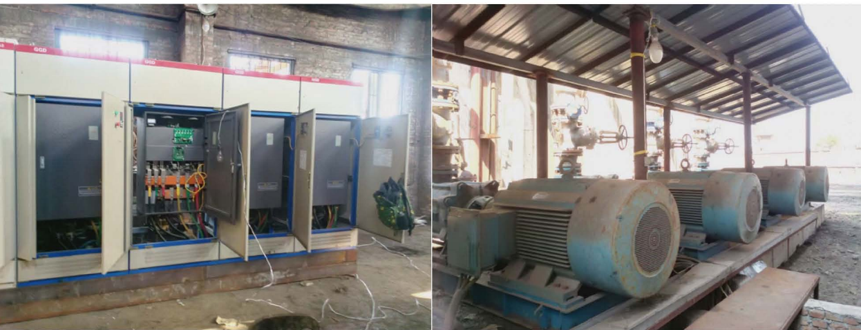
Easydrive 220kw inverters applied for steel mill
