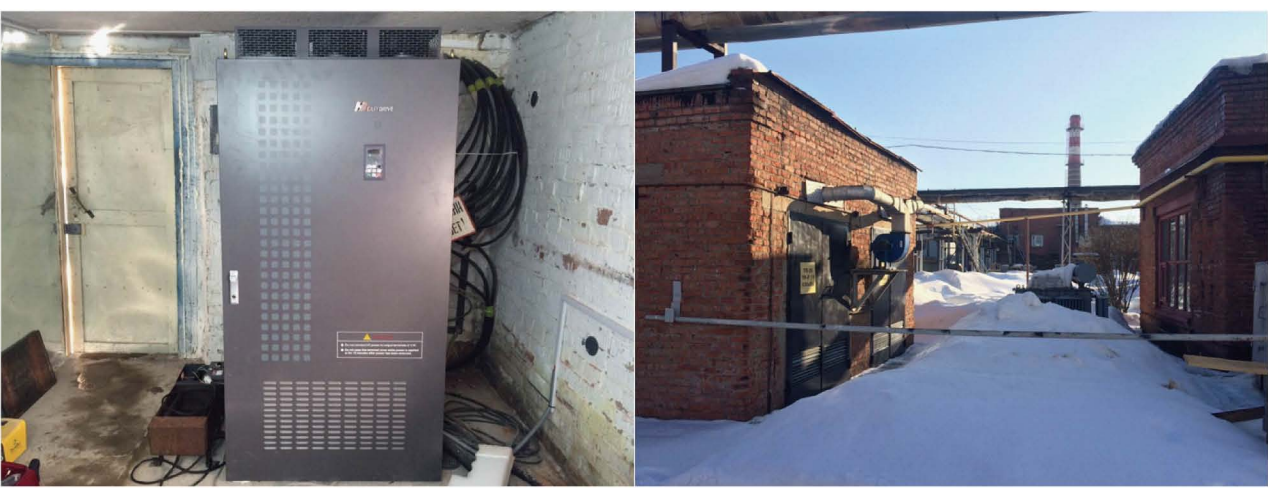
Easydrive 500kw inverter applied for centrifugal fan
