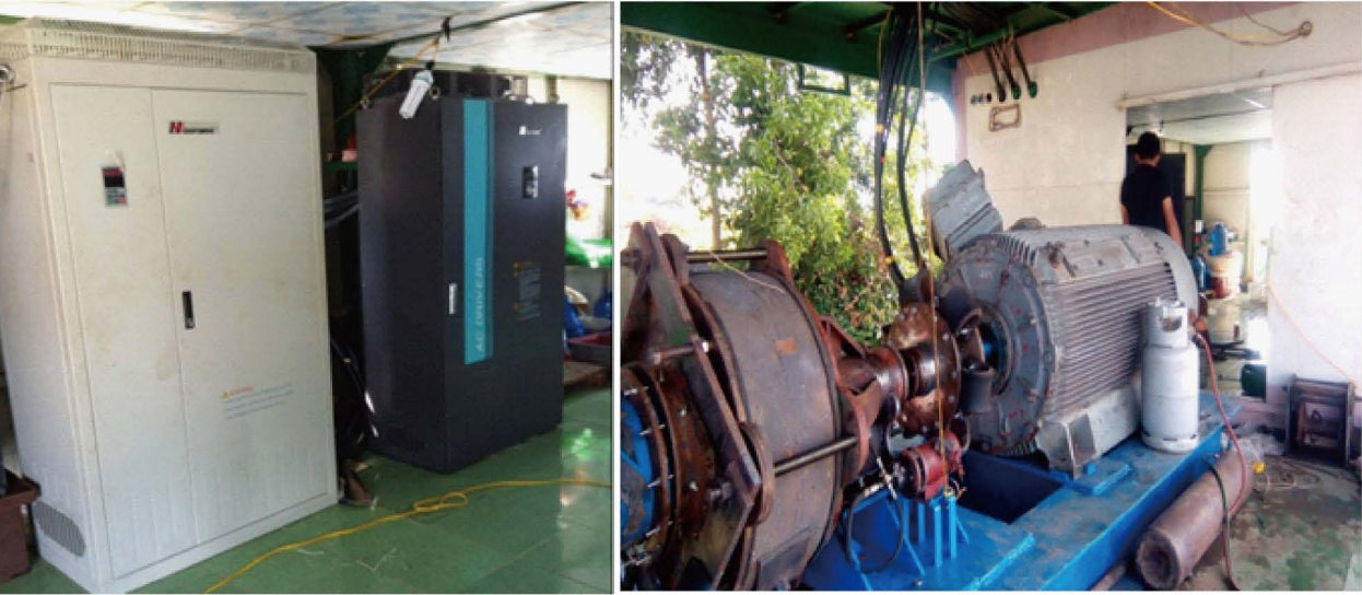
Easydrive 160kw inverters applied for circulating water pump
