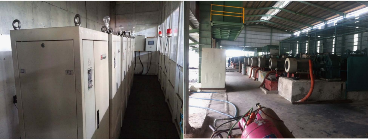
Easydrive 220kw inverters applied for steel mill
